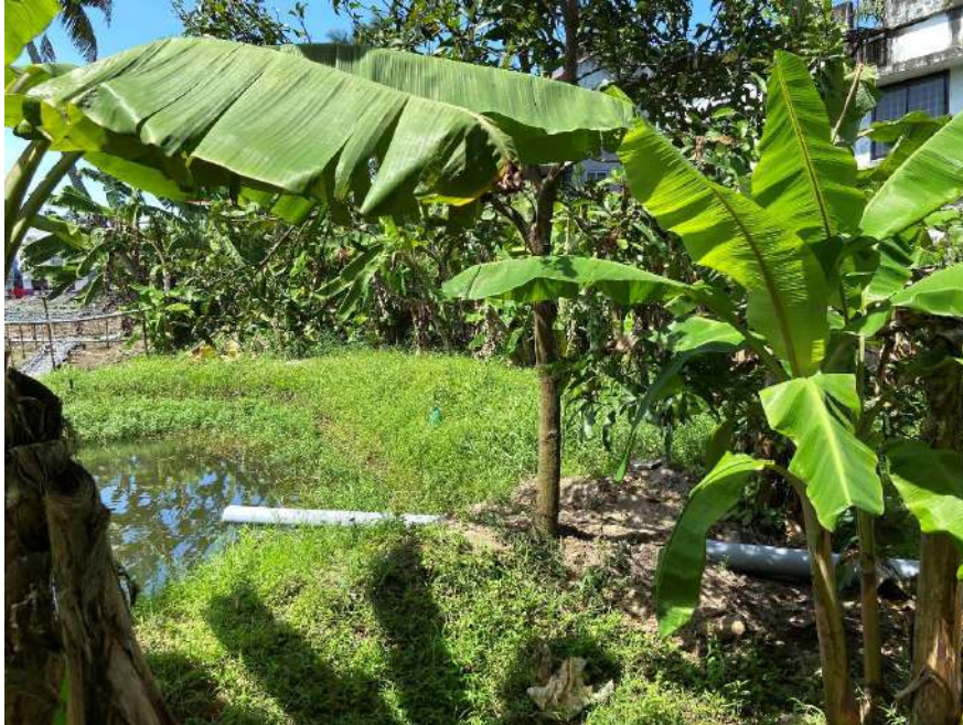
Pic of Rainwater harvesting unit
