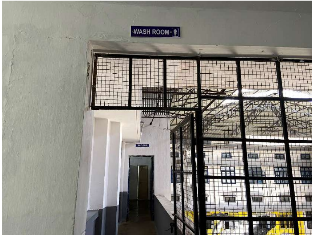
Pics of Toilets from doorway
