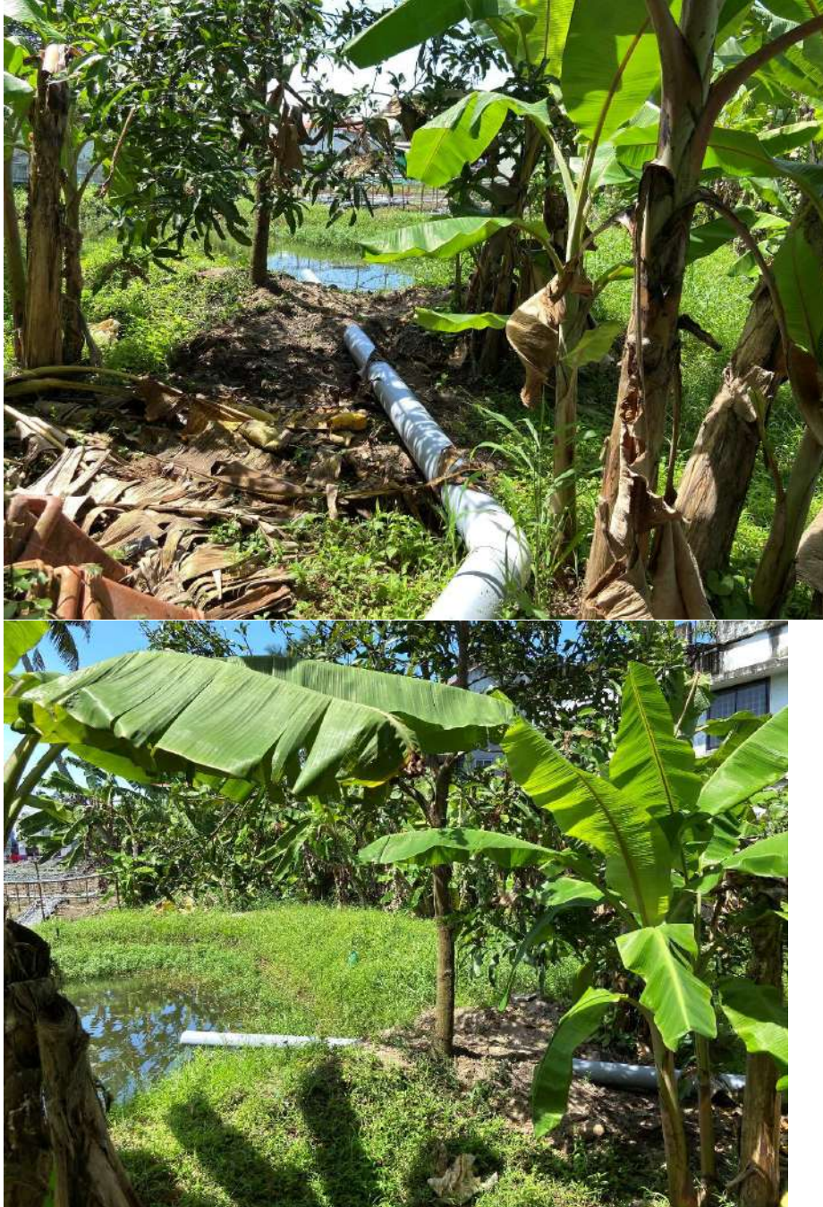
Pic of Rainwater harvesting unit
