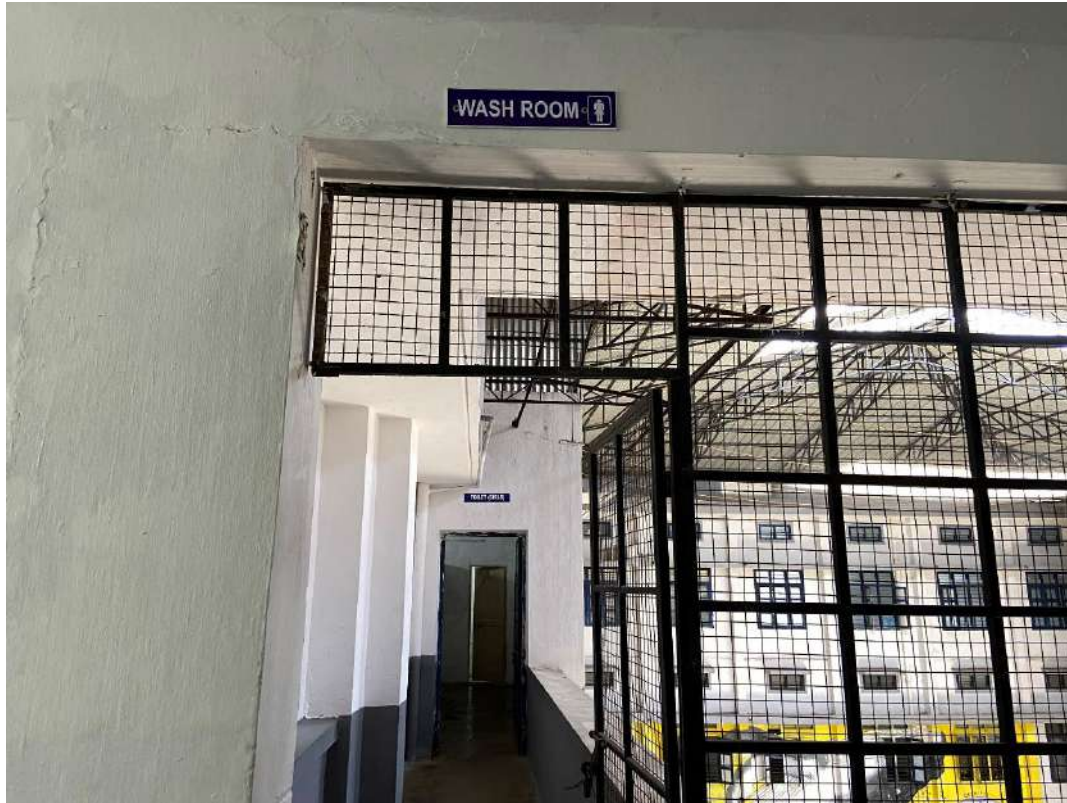
Pics of Toilets from doorway
